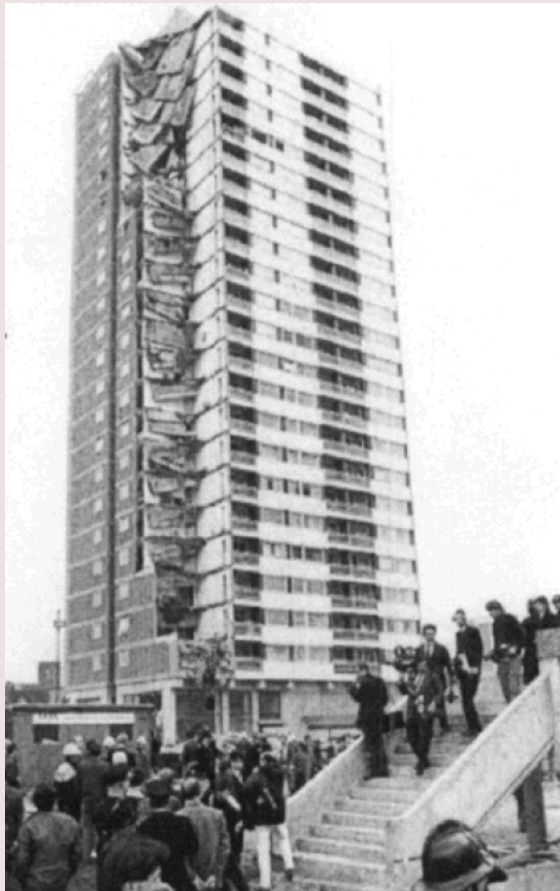
Ronan Point Collapse - 1968
